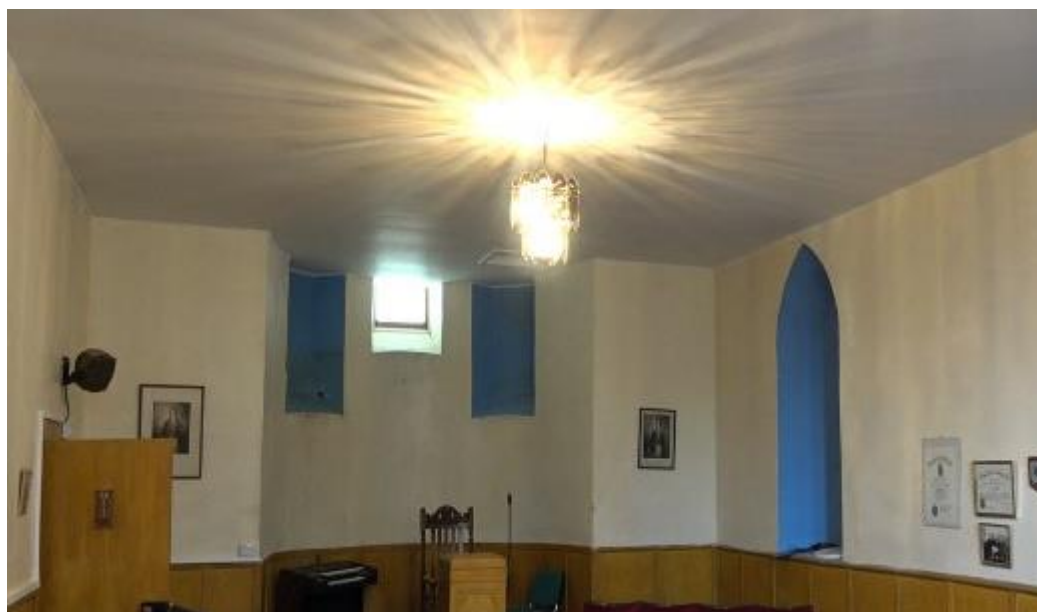
The new ceiling in Lodge Loch Ewe
